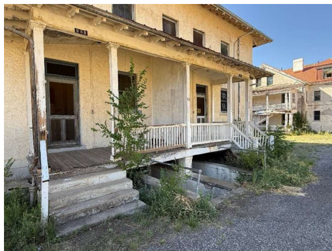
Building 53, Rear Porch
